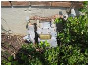
Acceptable Main Gas Valve: Located at gas meter
