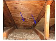
18. Main Attic Sheathing: Plywood - Poor repair at 2 areas near ridge at rear slope - No H clips installed and repair only spanned one truss - Recommend additional support be installed
