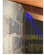
Marginal Sheathing: Plywood - Water stains and slight damage present, Areas of sheathing have been repaired
