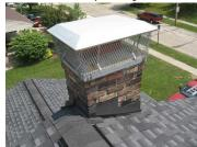
Acceptable Chimney Flashing: Galvanized
