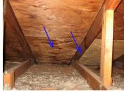
Acceptable Ventilation: Ridge and soffit vents Acceptable Insulation: Fiberglass loose fill
