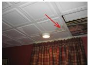
Acceptable Ceiling: Suspended Acoustical System - Evidence of past water staining
